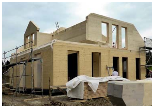
Moisturesafe and thereby sustainable buildings
